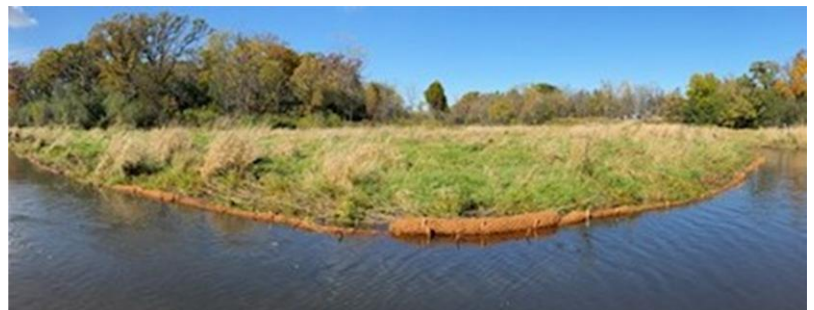
Bio-logs were installed on a significant stretch of Whitewater Creek’s bank.
