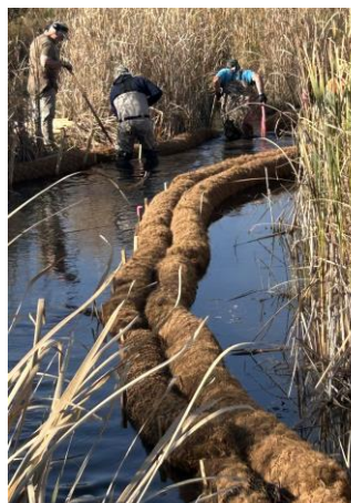
SEWTU & OBTU Teaming to install Bio Logs in Tichigan Creek
