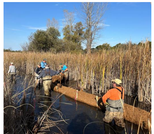
SEWTU & OBTU Teaming to install Bio Logs in Tichigan Creek
