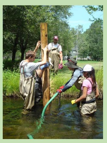
Campers operating the high pressure water jet drill to sink pylons deep into the stream bed.
