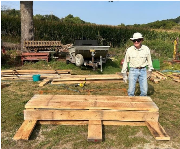
Willie admires a lunker structure constructed by our OBTU team. The lunkers were built with very heavy oak & walnut harvested by the DNR from the Yellow River State Forest.
