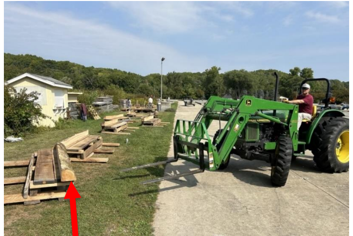
The new design features a quarter log mounted on the stream-facing top to reduce the washout of rock and sod that will be placed over the top of the structures to stabilize the bank. Mike Siepker, Iowa DNR, drives a tractor to move the heavy lunkers constructed at the Decorah fish hatchery.
