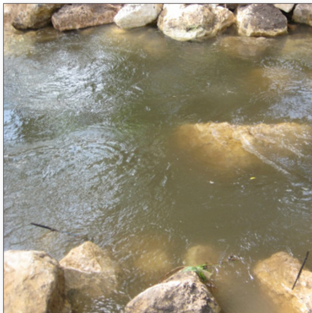
Farmers Valley Creek is narrowed to its original size and flow velocity in this location.
