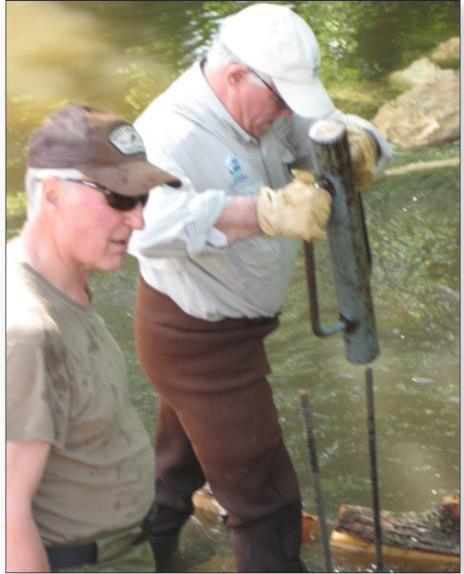
Dave Luardini drives rebar into the stream bed while Greg Prosen assists.
